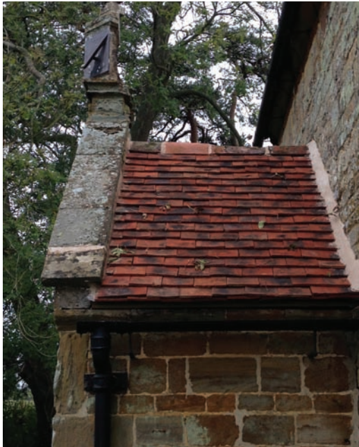
Porch at St John the Baptist, Plumpton
