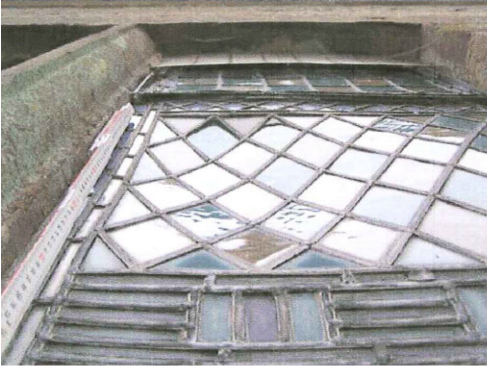
Greatworth – windows restoration – before and after
